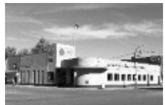
Streamline Moderne bank building
