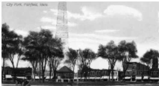
Central Park, July 1910. The six electric arc lamps at the top of the 185 foot tower had to be changed daily; kids clamored to help. Dismantled in 1910. Viewed from the southeast corner of the square.
