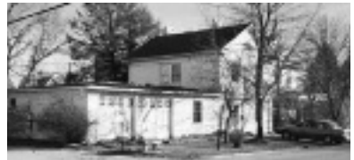
R. B. & Lizzie Loudon House, here showing the Loudon garage doors.
