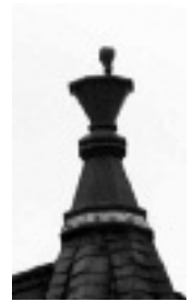
Mortar and pestle finial detail.
