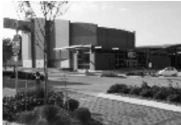
The Stephen Sondheim Center for the Performing Arts, southern wing of the Fairfield Arts & Convention Center.
