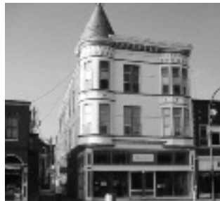
Queen Anne commercial building on the north side of the square.
