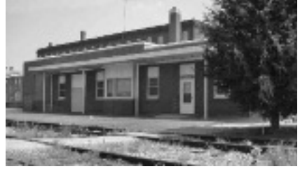
Former Rock Island Train Station
